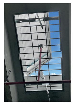
When the grid needs to meet ANIA requirements, it is made with 15mm diameter iron rods and a mesh size of 150x300mm.
