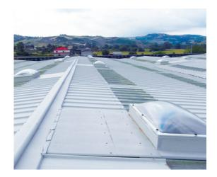
Curbs, to be assembled on-site, for coupling with double-slope roofs made of straight corrugated sandwich panels. These curbs can be positioned with either the short side or the long side parallel to the ridge. They are constructed with a C-shaped section of steel sheet with chromatic finishes. The height and insulation panel in polyurethane can be customized according to project requirements.
